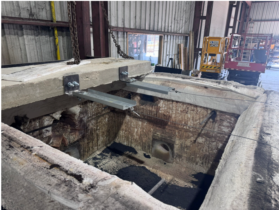
Photo No. 6 Assembly Positioned into Furnace Prior to Test 1
