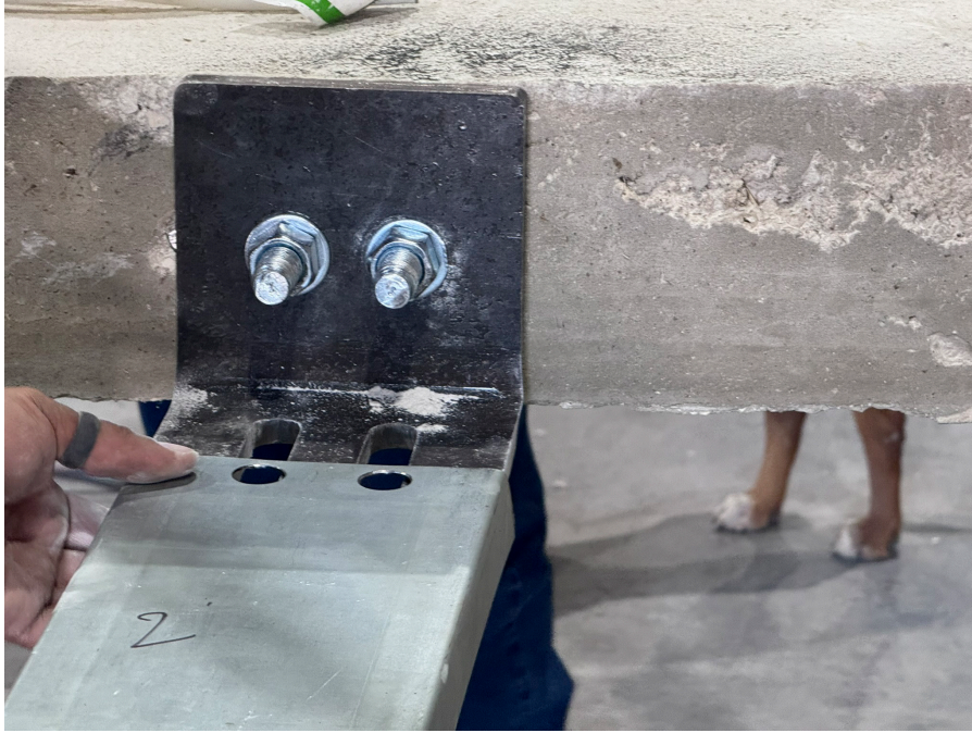
Photo No. 3 U- Channel Connected to Connector
