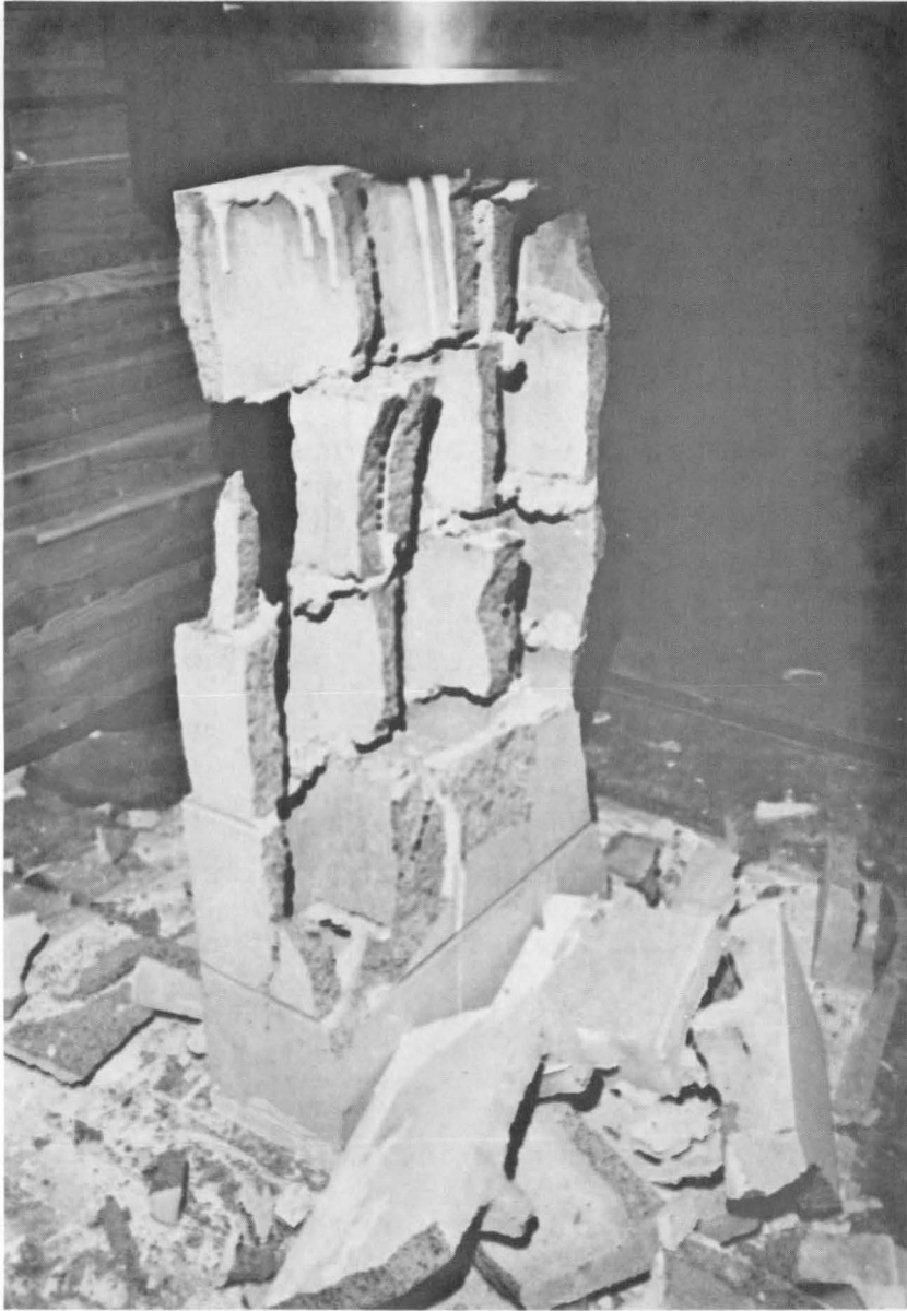
PLATE 1 Web Misalignment in Running Bond Construction
